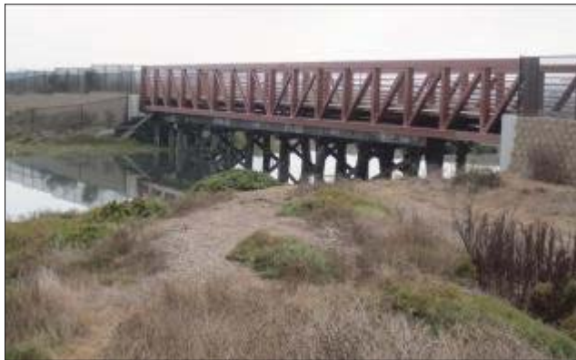
New bike path bridge built over an old train trestle. Photo: John Blocker.
