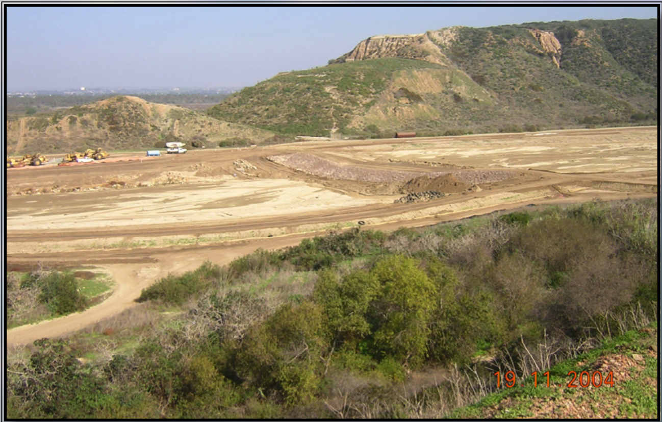
Goat Canyon before sedimentation basins had enough riprap to stabilize the berms; photo taken just after the Nov. 2004 deluge.
