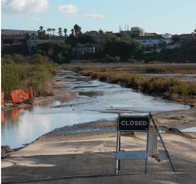
Sediment-laden stormflow crosses non-elevated park entrance road effectively smothering 18 acres of salt marsh in 2005.
