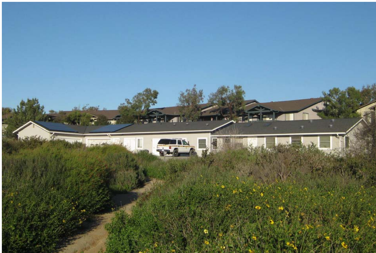
Operations Building (Garage, Lab and 2007 Operations Building) Note rooftop sustainable design features: Solar Tubes for daylight office lighting and Solar Panels for energy generation.
