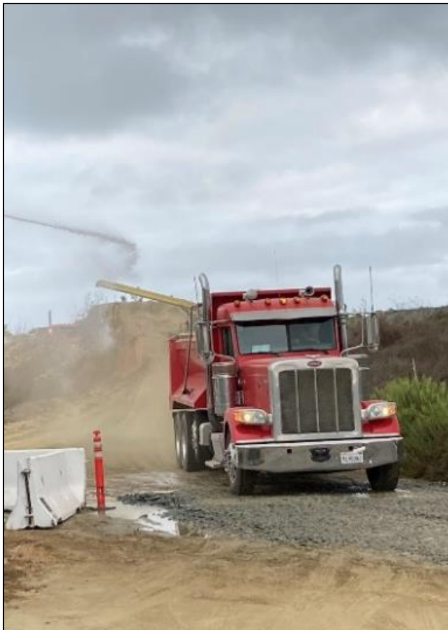
Sediment transported to beneficial reuse or disposal via truck requires best management practices including tracking controls, load coverings, and limited operational hours.
